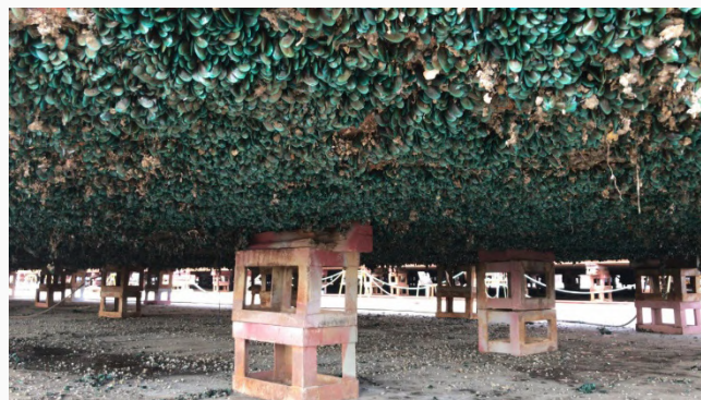
Figure 1. Bottom surfaces with biofouling growth
